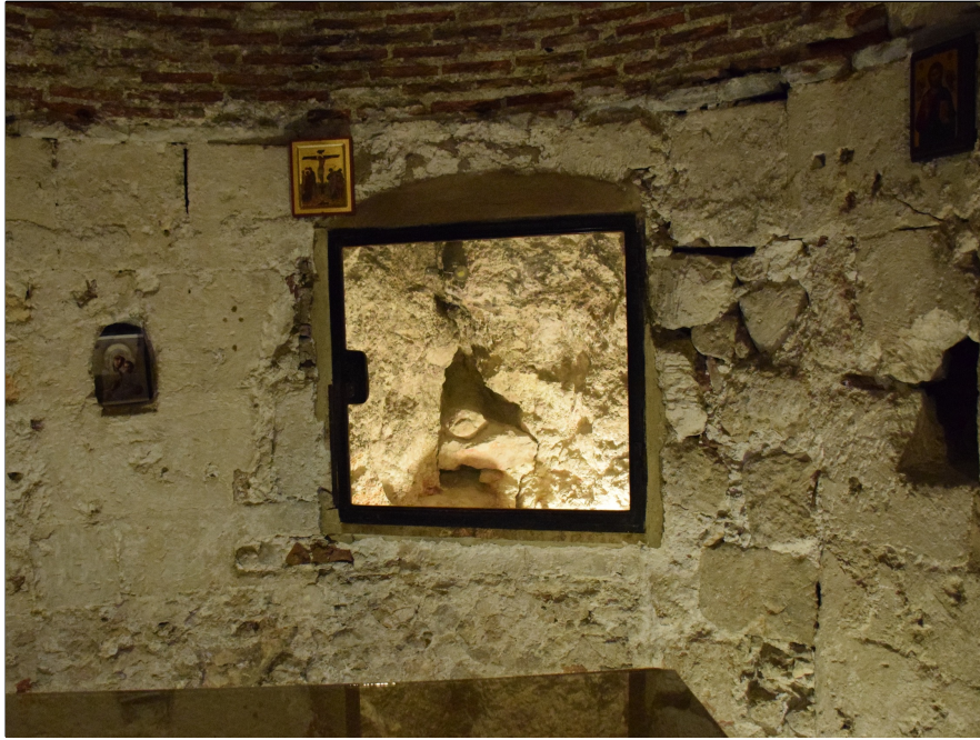
Traditional crack that formed with the earthquake upon the death of Jesus (Matt 27:51). This is downstairs under "Golgotha." (January 2020)
